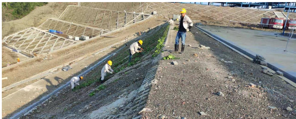
Protection of original soil and vegetation by solidification via concrete shotcreting
