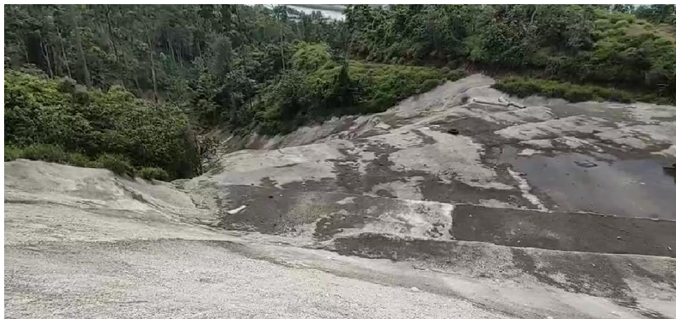
Protection of original soil and vegetation by solidification via concrete shotcreting
